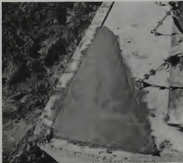
FIG. 4. COMPLETED CORNER FULL SIZE PANEL
